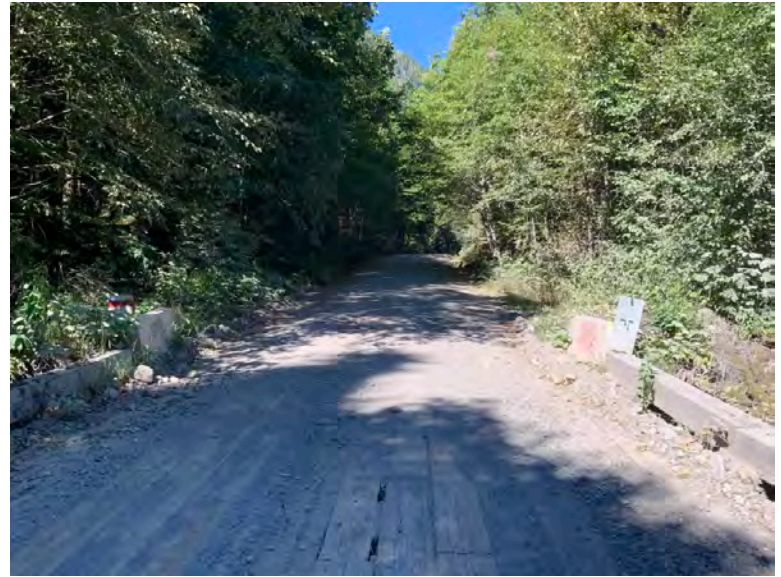
Approach from Right Bank when facing downstream
