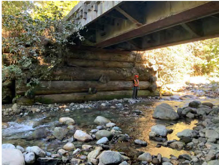
Right Bank Abutment when facing downstream
