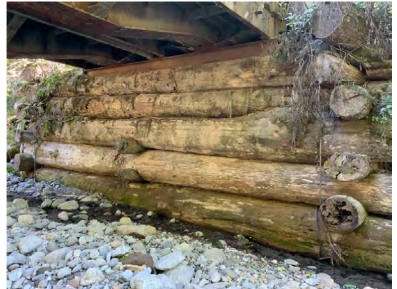
Left Bank Abutment when facing downstream
